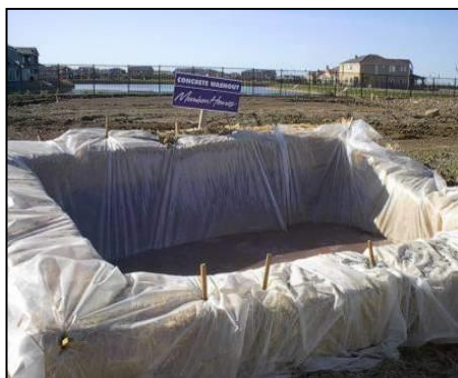
Plate 3-1 Typical concrete wash out areas
