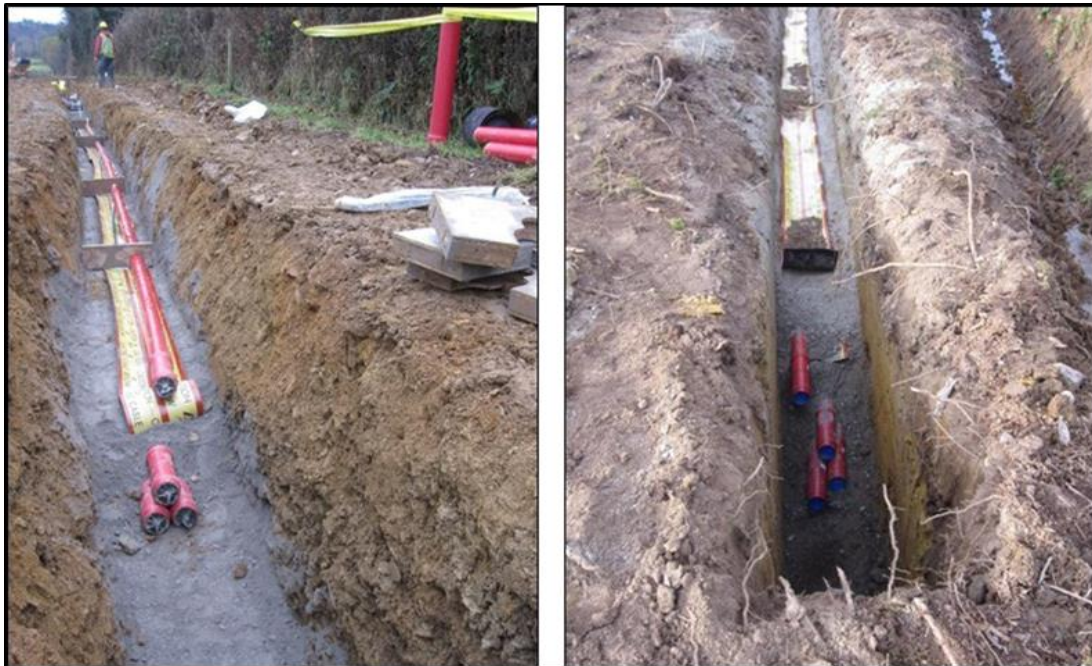
Plate 2-1 Typical Cable Trench View
